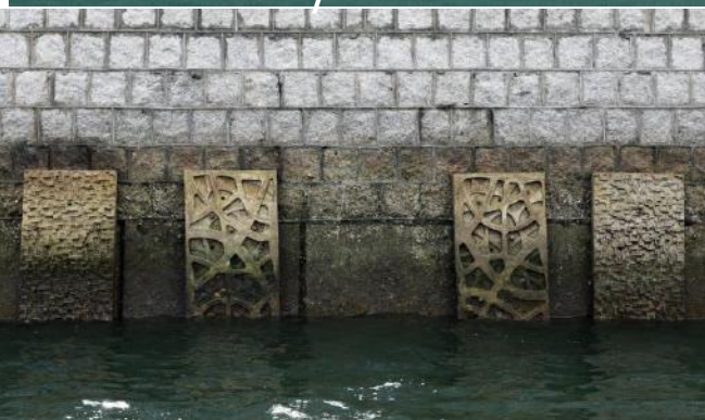
Use of locally-manufactured eco-materials at Pier Foundation
